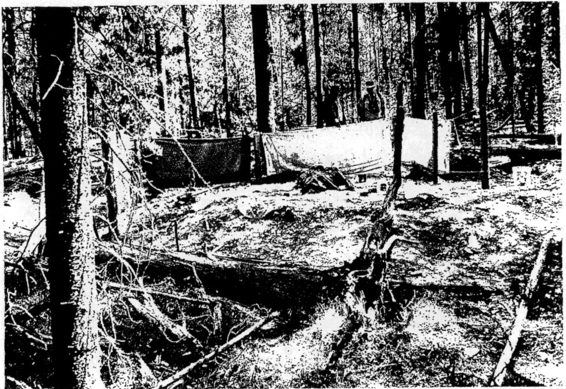
Fig. 13. Large "Septic Tank" Latrine
