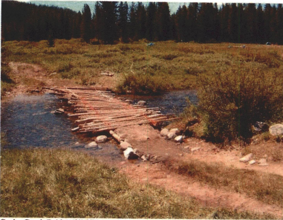
Cache Creek Bridge 6/16/01
