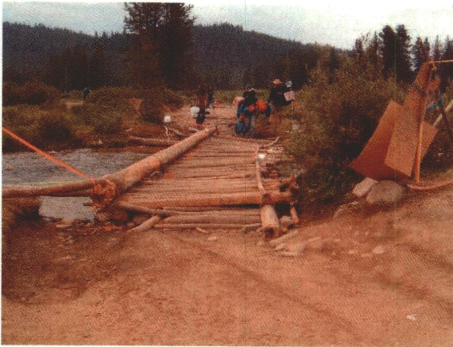
Cache Creek Bridge 7/7/01
